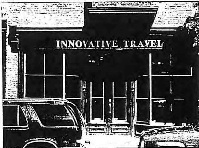
Appropriate: A flush-mounted wall sign is one that is mounted flat to the wall; in most cases, a flush-mounted wall sign should be positioned just above the display window.
