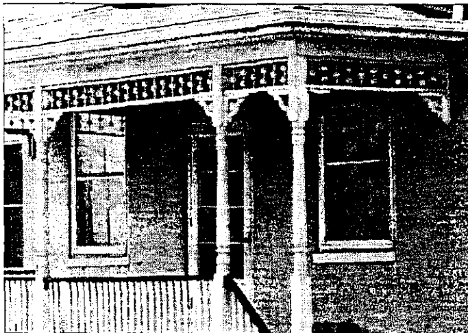
Similar architectural details (i.e. brackets, columns, jig-saw ornaments) should be incorporated in the design of an addition.
