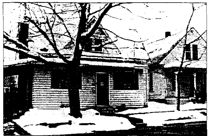
Do not enclose a historic front porch. A porch should remain open to the air. Compare the character of the enclosed porch on the left to that of an original porch on the home to the right.
