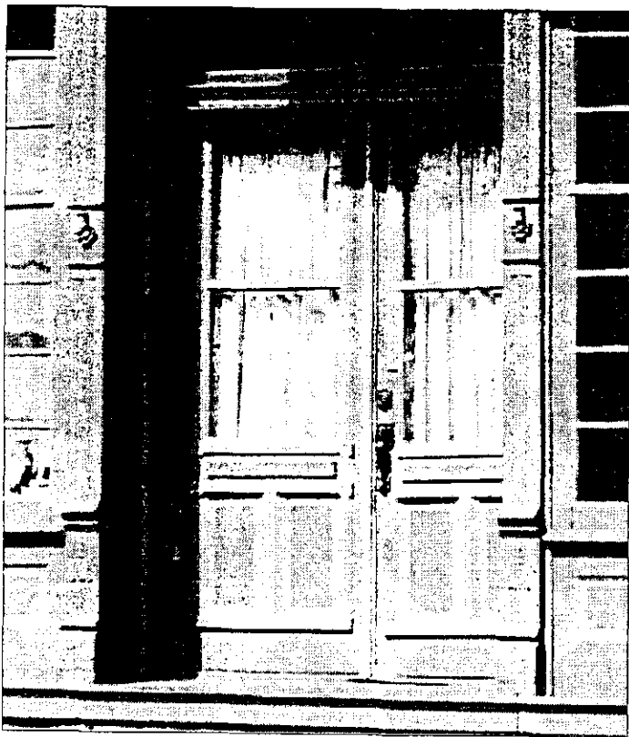
Preserve a historically important door when physical conditions permit. Preserve all significant features of a historic door, including: frames, sills, heads, jambs and moldings.
