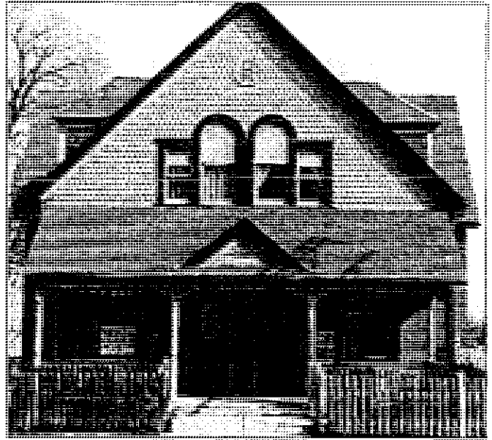
The Victorian era residential buildings in St. Charles, such as this one at 508-510 South Main Street, incorporate many simplified characteristics of the style such as the jig-saw trim, the wall textures and the round-topped windows.
