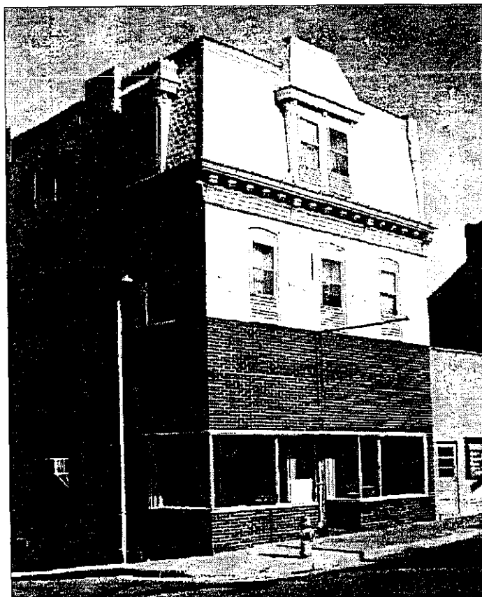
More recent alterations, additions or new construction that are not historically significant may be removed. For example, the more recent ground floor alterations to this building in Washington, Missouri, have no historic value. Reconstruction of the original design would be preferred.
